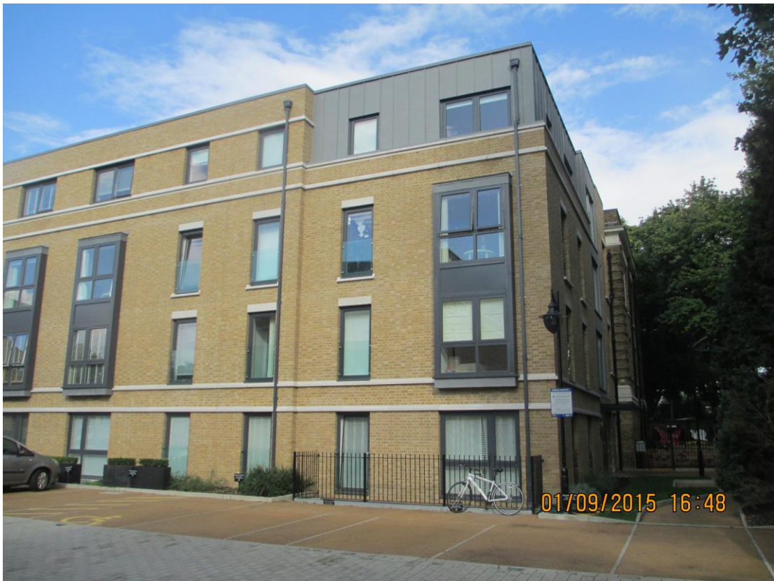
Image 3 – Lightwell in context with existing building.
